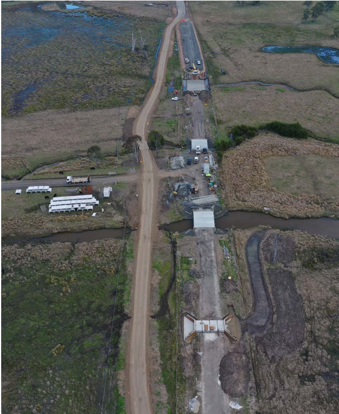
Work on the Clarence Way upgrade project continued throughout 2024-2025 and included flood immunity projects at Culmaran Creek, pictured, and Tunglebung.
