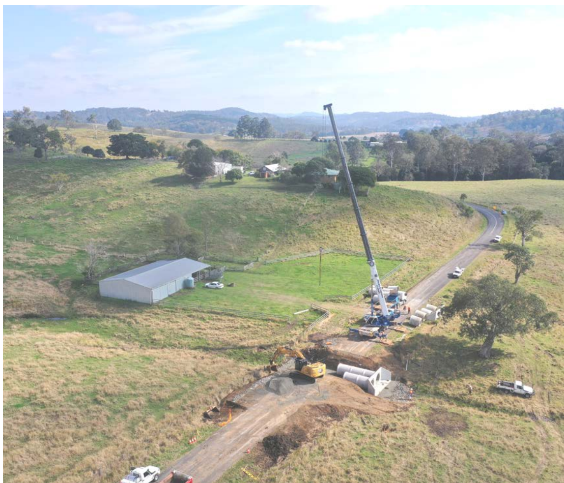
A crane lifts a pipe into place during a project to install a number of new culverts on Omagh Road.
