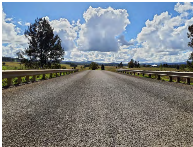
CZ3-S2 - COMPLETION PHOTO AT BEAN CREEK NO. 1 BRIDGE
