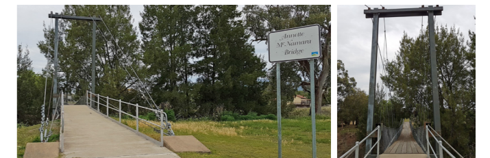
Opportunity for a future connection using a swinging pedestrian bridge (example from Annette McNamara brige in Quirindi)
