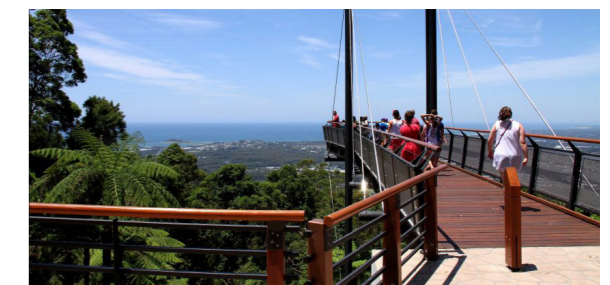
Example 'skywalk' at Sealy Lookout, Coffs Harbour (photo by Coffs Coast)
