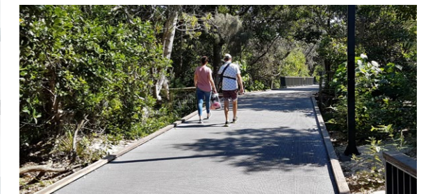
Example of a boardwalk made from FRP composite material
