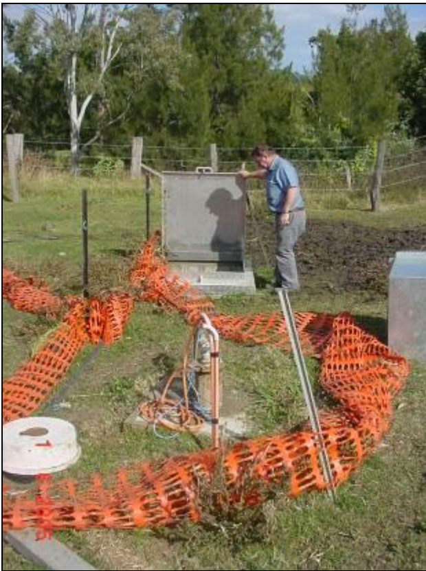
Photos of Kyogle Bore No.1 after commissioning. Note stock proof fencing still to be installed, and additional valve work installed to allow for pumping to the adjacent football ovals.
