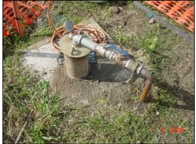
Photos of Kyogle Bore No.1 after commissioning. Note stock proof fencing still to be installed, and additional valve work installed to allow for pumping to the adjacent football ovals.
