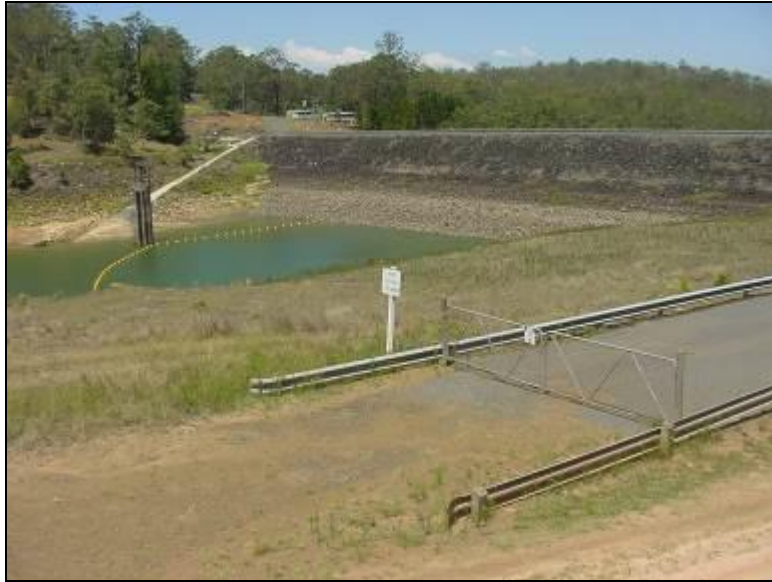
Toonumbar Dam during drought in December 2002. Note extension of boat ramp constructed due to extremely low water levels This is indicative of the water level the dam would be at When Council would have access to the 240ML dead storage
