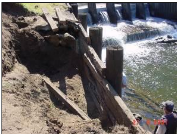
Weir during restoration works in 2001 following flooding earlier in the year
