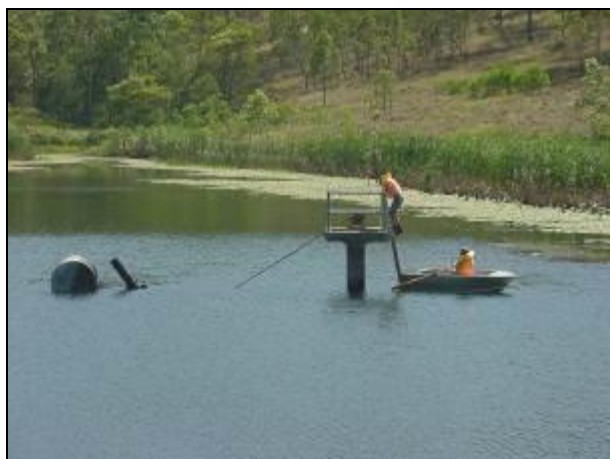
Accessing the trunnion winch, note intake Trunnion above water level to allow inspection Of the internal pipe work through the dam wall
