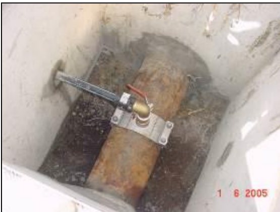
Photos of Kyogle Bore No.1 after commissioning. Note stock proof fencing still to be installed, and additional valve work installed to allow for pumping to the adjacent football ovals.
