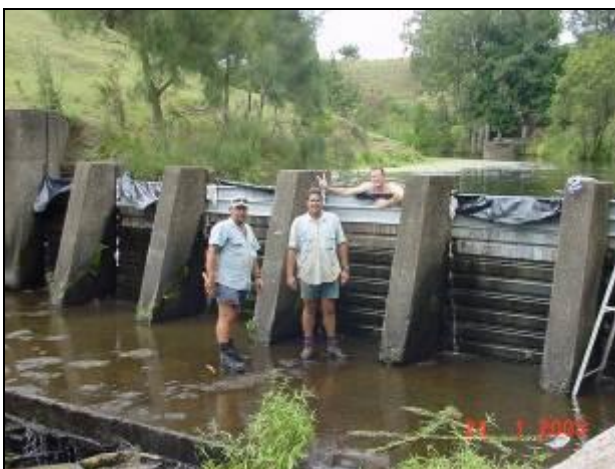
The weir following works to eliminate leakage including plastic lining the upstream side
