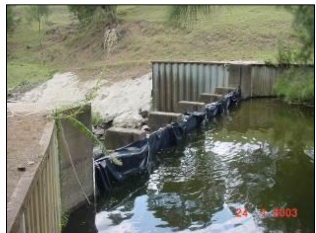
The weir following works to eliminate leakage including plastic lining the upstream side
