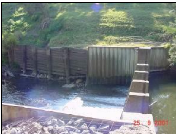
Weir during restoration works in 2001 following flooding earlier in the year
