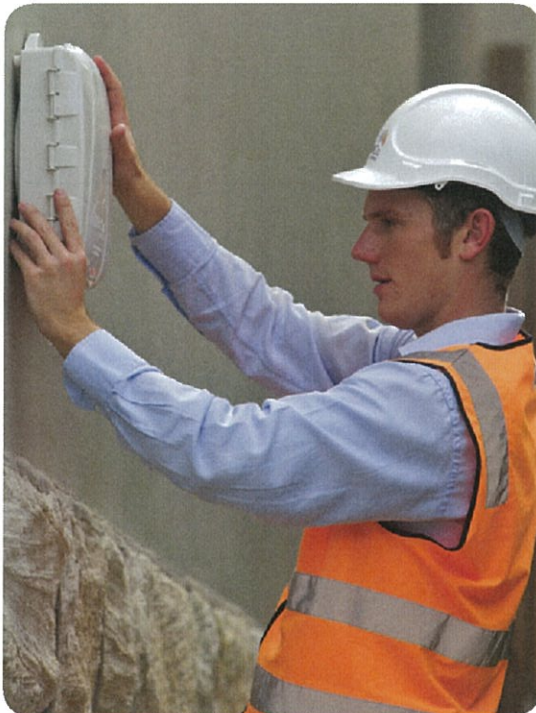
NBN Co or an NBN Co subcontractor will install fibre infrastructure to each premises in a new estate.
