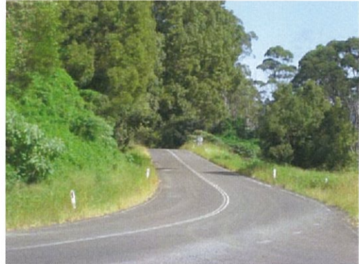
Typical lane width between Cawongla and MR142
