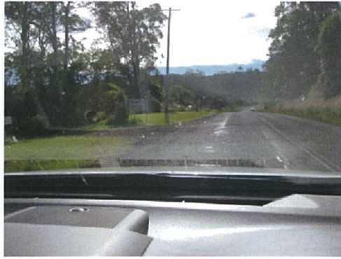
Looking north approaching café access on left
