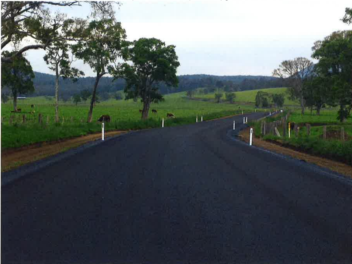
Photograph - Section of Mount Lindesay Road Upgraded in March 2015
