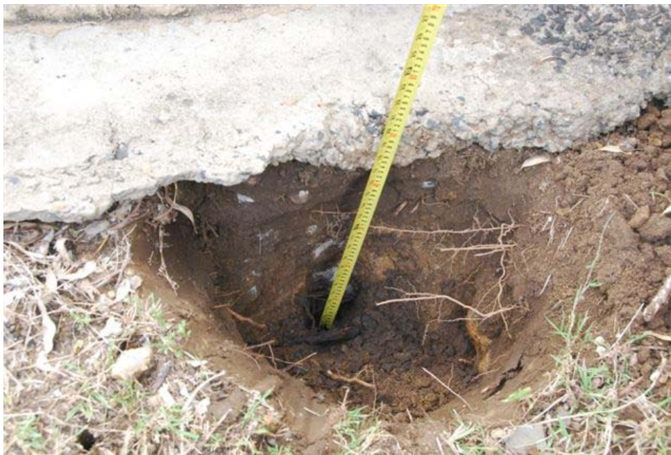
Photo 6.2 – Base of footing at bottom of tape bearing on moist topsoil
