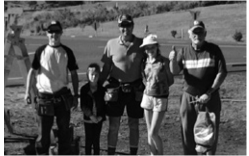
Long-time Council volunteer Bob Olive gives the shade shelter and barbecue area in Aboody Park Wiangaree the thumbs up during the construction.
