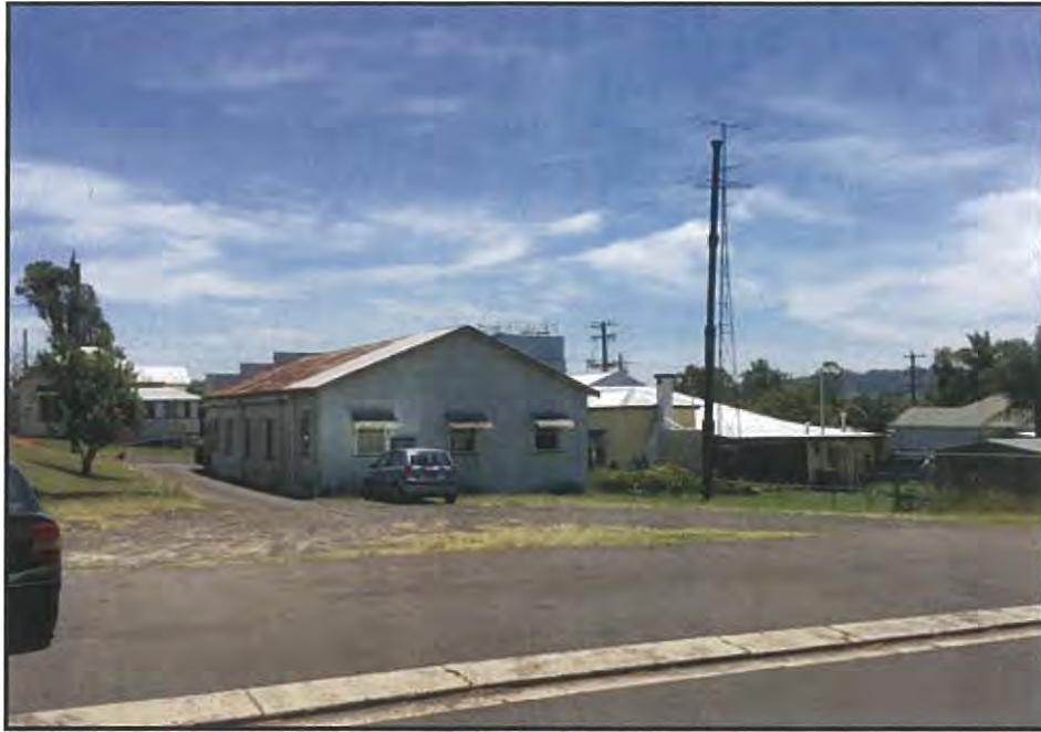
Works Depot Shed Adjacent to Development Site
